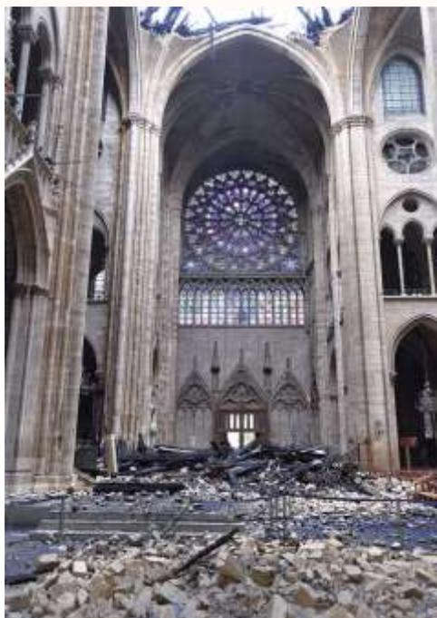
Debris inside Notre Dame after the catastrophic fire; the rose window appears to be intact, but the glass may have suffered from micro-cracks, requiring time-consuming repairs Photo: Bastien Louvet/SIPA/REX/Shutterstock; © 2019 Shutterstock
